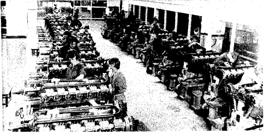
Liberty V-12 aircraft engines being produced by the Dayton-Wright Airplane Company in July 1918. (Note that women worked in the aviation industry during World War I as well as World War II.)
