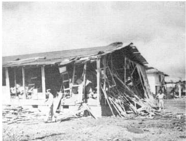
Russell J. Tener (left) and his friend Bill Enos (far right), while on guard duty at this PX warehouse, escaped harm when the building was shattered from the concussion of a bomb which left a crater (partly visible in left foreground) about 20 feet in diameter and 5 feet deep. (Russell J. Tener)
