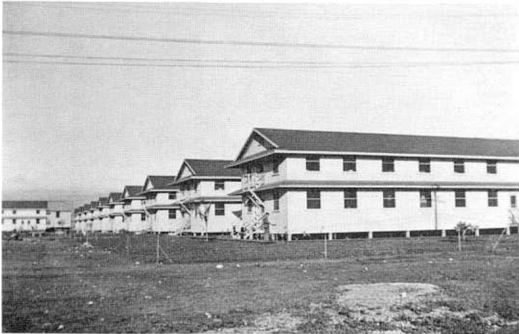
Above, the wooden barracks of “Splinter City” at Hickam Field, 1940-1941. (Bernard C. Tysen)
