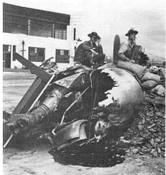
Another gun emplacement, hastily constructed in front of Hangar 5, was manned shortly after the raid by PFC Raymond Perry (left, with binoculars) and Cpl Howard Marquardt of South Dakota. A burned-out aircraft engine, sand bags, table, and debris from the attack made up the construction material for this bunker.
