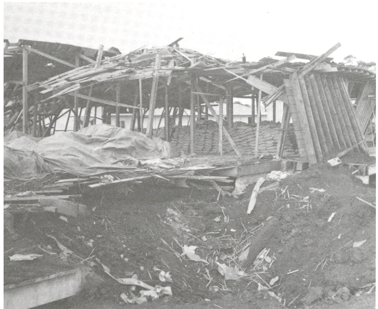
Splintered building filled with bags of cement. (Joe K. Harding)
