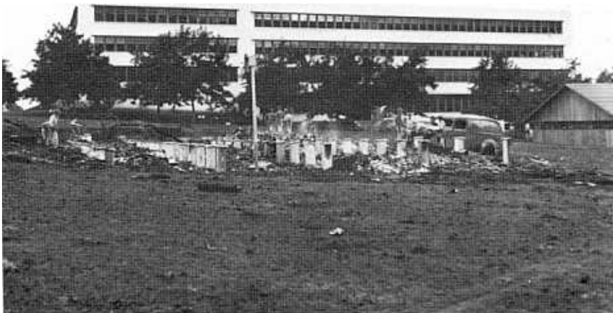
Wheeler personnel inspect what remained of a building site following the 7 December 1941 attack. The new barracks stands on an embankment in background.
