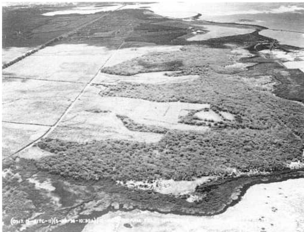
Aerial view of what was originally known as Tracts A and B, acquired on 3 April 1935 at a cost of $1,095,543.78 for the construction of Hickam Field.
