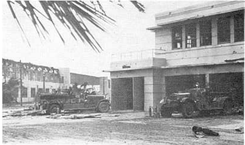
The Hickam fire station, wrecked by bombing and machine-gun fire.
