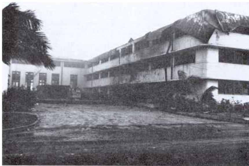
Wing L of Hickam Field's big barracks, with its fire-blackened, bullet-scarred walls and wrecked roof, was devastated by the attack. Mess hall is at left.
