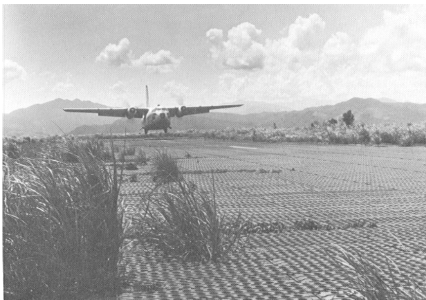
Pierced steel planking forms a runway at a remote outpost, dependent on C-123 deliveries, 1966.
