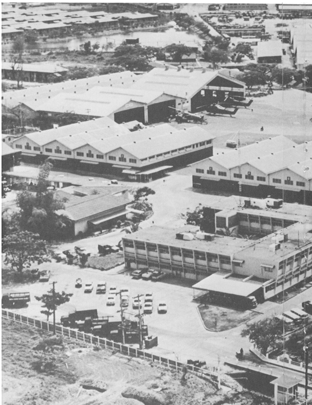
Air America headquarters, Udorn Air Base, Thailand.
