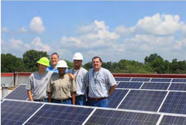
Students from the Shreveport Job Corps Center pose proudly next to the solar panels they helped install on the roof of a campus building.
