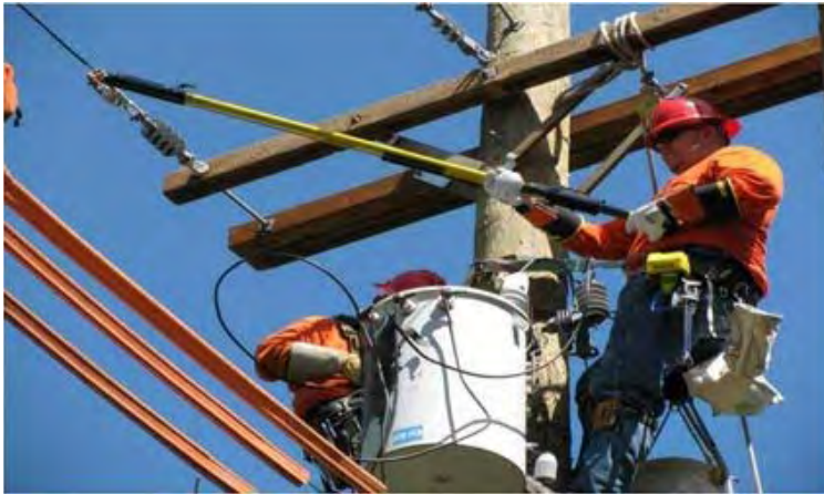
Overhead Line Construction students from the Oneonta Job Corps Center practice their skills at a special training facility near campus.
