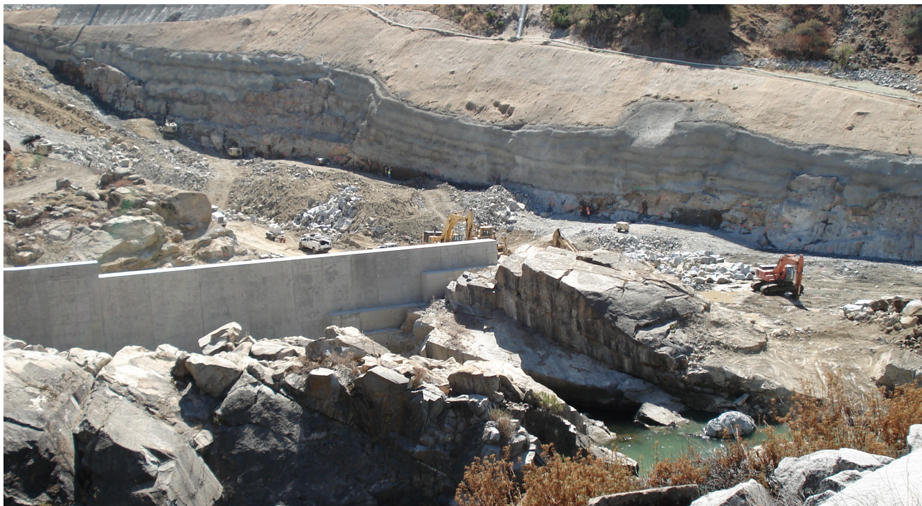
A view of the new spillway construction at Folsom Dam
