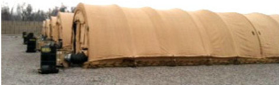
Pictured above is the Alaska Small Shelter System attached to one of the tents at the Transit Center at Manas, Kyrgyzstan. The fly, which goes over the top of the tent, helps block the sun in the summer and the wind in the winter. An insulated liner on the inside of the tent helps regulate the temperature year-round.
