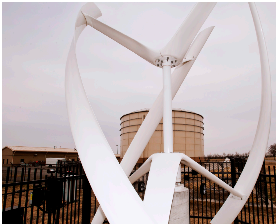
A wind turbine slowly rotates on a calm day at McConnell Air Force Base, Kan. The turbine, currently the only one on base, generates power for the 22nd Civil Engineer Squadron utility shop, pictured behind the turbine. The performance and benefit from this turbine is being studied to determine if more could be implemented around base. (U.S. Air Force photo/Airman 1st Class Victor J. Caputo)
