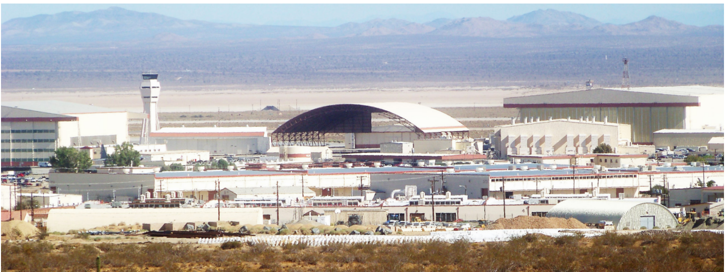
After an extensive review of eight years of utility bills at Edwards AFB, Calif., The Utility Rates Management Team at the Air Force Civil Engineer Center, Tyndall Air Force Base, Fla., discovered the Air Force was due a refund of nearly $3.7 million. (U.S. Air Force photo/Ms. Jennifer Elmore)
