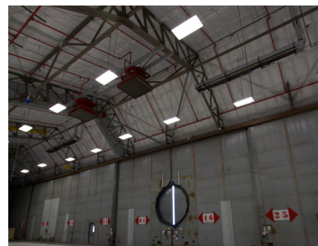
Bottom right: T-8 lights and digital controls in a hangar at Pease ANGB, N.H. (U.S. Air Force photos/Eddie Green)
