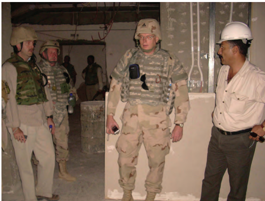
Iraqi construction supervisor guides U.S. contractors through hospital under construction in Basra
