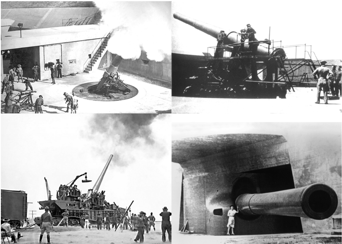
Major types of armament emplaced at Fort MacArthur: 12- inch mortar (upper left); 14- inch disappearing carriage rifle (upper right); 14- inch railway gun (lower left); and 16- inch rifle (lower right). (Photographs courtesy of Fort MacArthur Museum)
