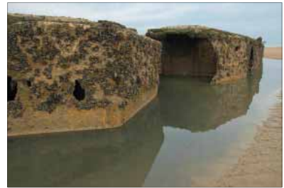
Above: Crumbling concrete pontoons encrusted with mussels lie on the beach at Arromanches, France. Now a reminder of the Mulberry Harbor complex built to offload troops and supplies, the hulks sit on Gold Beach not far from the D-Day Museum.
