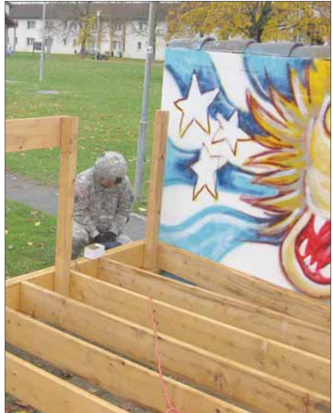
Technical Engineer Staff Sgt. Robert Owens with the 18th Engineer Brigade and a native of Hornbeck, La., uses a power drill to assemble the deck frame for the Lion's Den on Patrick Henry Village in Heidelberg. Staff Sgt. Shaun Emmett
