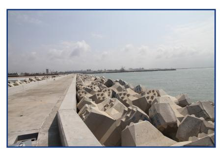
The extended sand-stopping jetty ensures that sand does not enter the port entrance channel and reduces maintenance costs, estimated to save the port over \$2.1 million annually.
