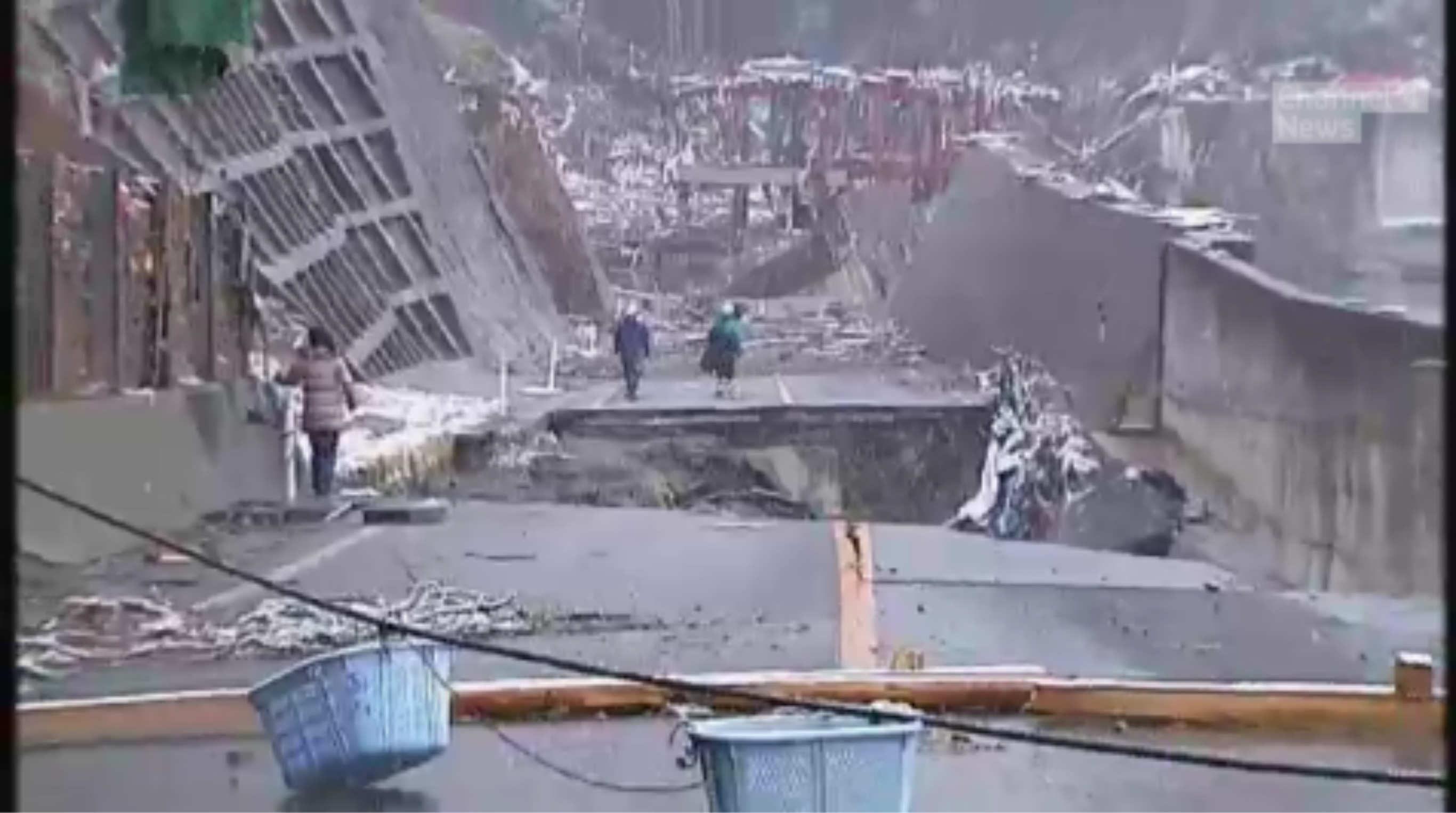
Kamiashi City Seawall
