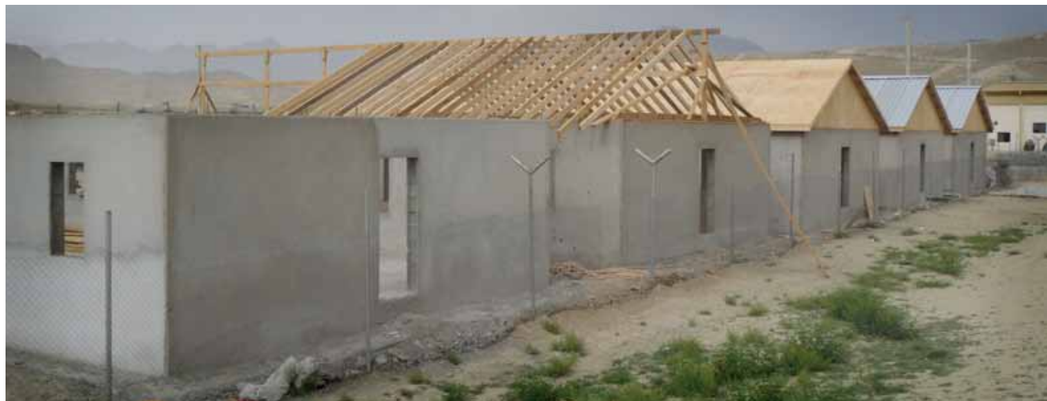
B-huts under construction at Kabul Military Training Center.
