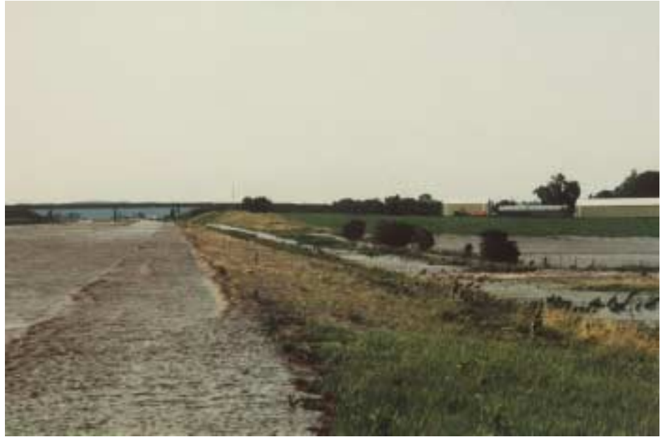
Figure 2. Overflow on Interstate 29 near Hamburg, Iowa, on June 17, 1998. Water over Interstate 29 was about 0.5 foot deep and 1,775 feet wide; measured rate of overflow was 712 cubic feet per second.
