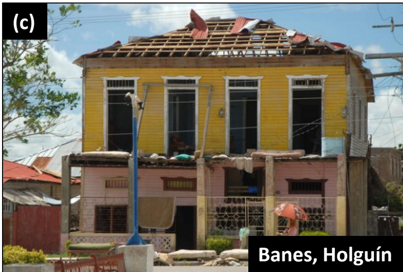
Figure 28. a) House in Holguin destroyed by Sandy's strong winds, b) severe structural damage in Holguin, c) roof damage to a residence in Holguin, and d) storm surge flooding at the Hotel Baconao near Santiago de Cuba. Images courtesy of the Cuban Meteorological Service.
