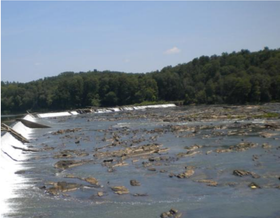
Figure 24. Augusta Diversion Dam and Shoals
