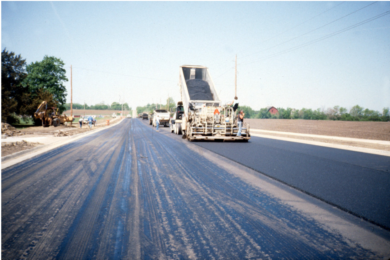
Figure 34. Photo. Streaking in spray application caused by improper pump pressure and/or spray bar height.
