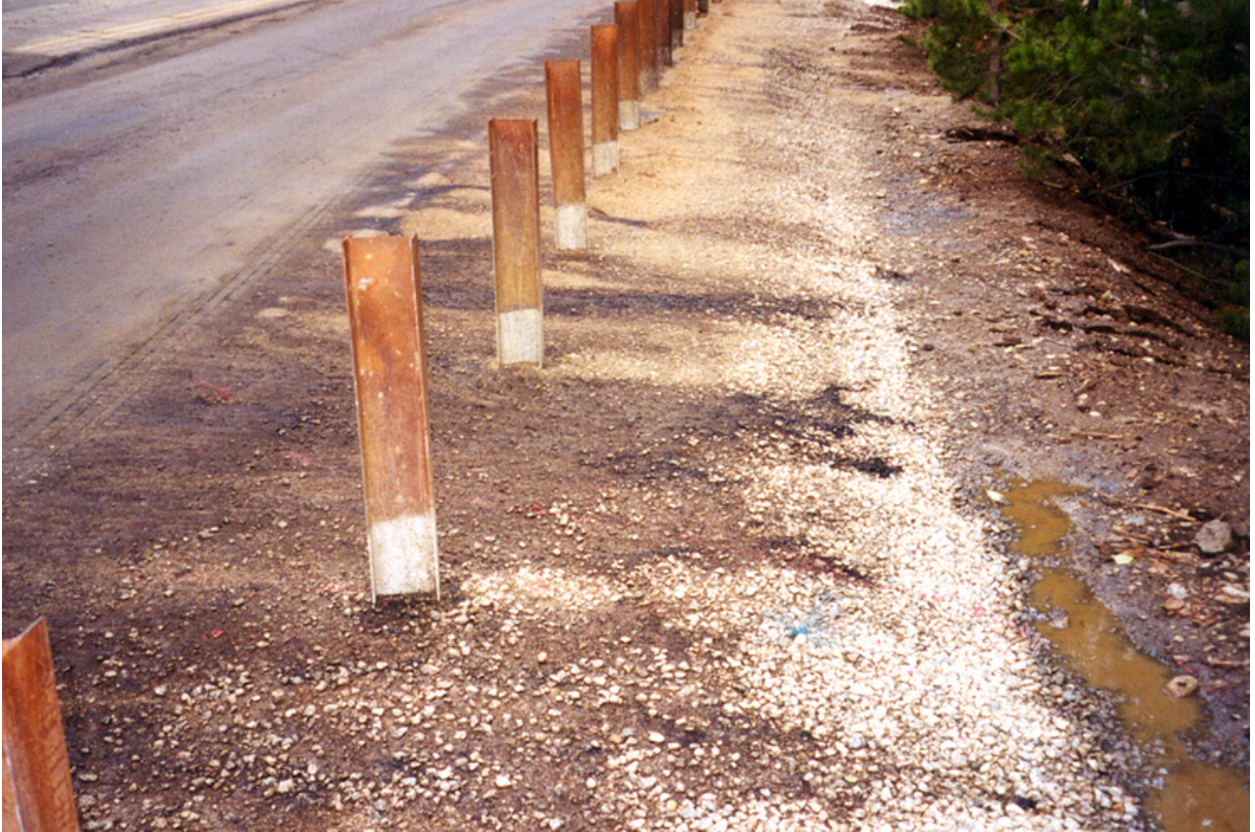
Figure 39. Photo. Prime runoff caused by rain shower on freshly applied prime.
