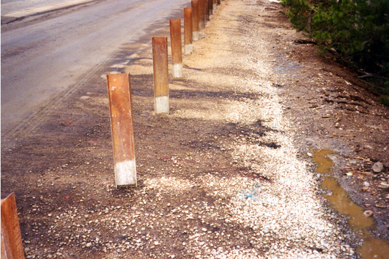
Figure 29. Photo. Effect of rain on a freshly applied prime coat.
