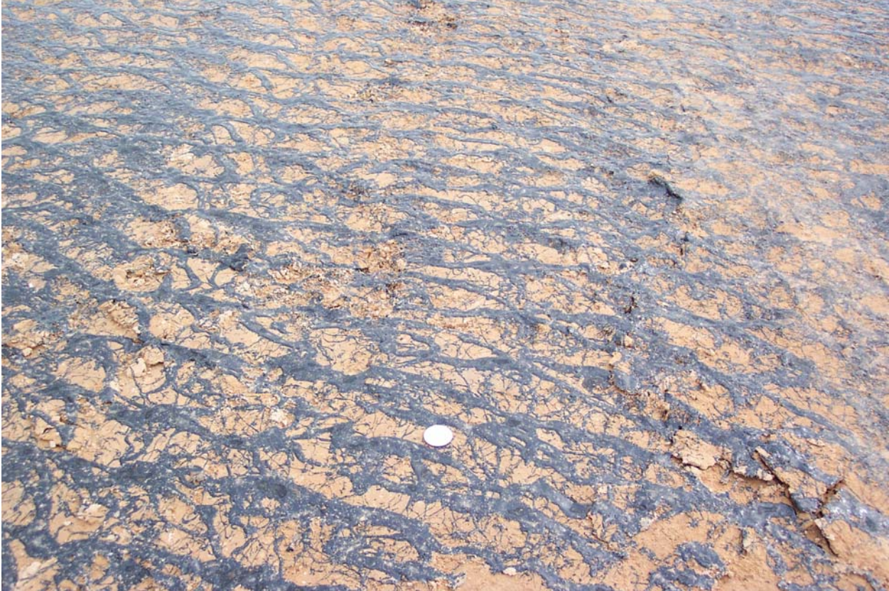
Figure 4. Photo. Prime applied at too high a viscosity.
