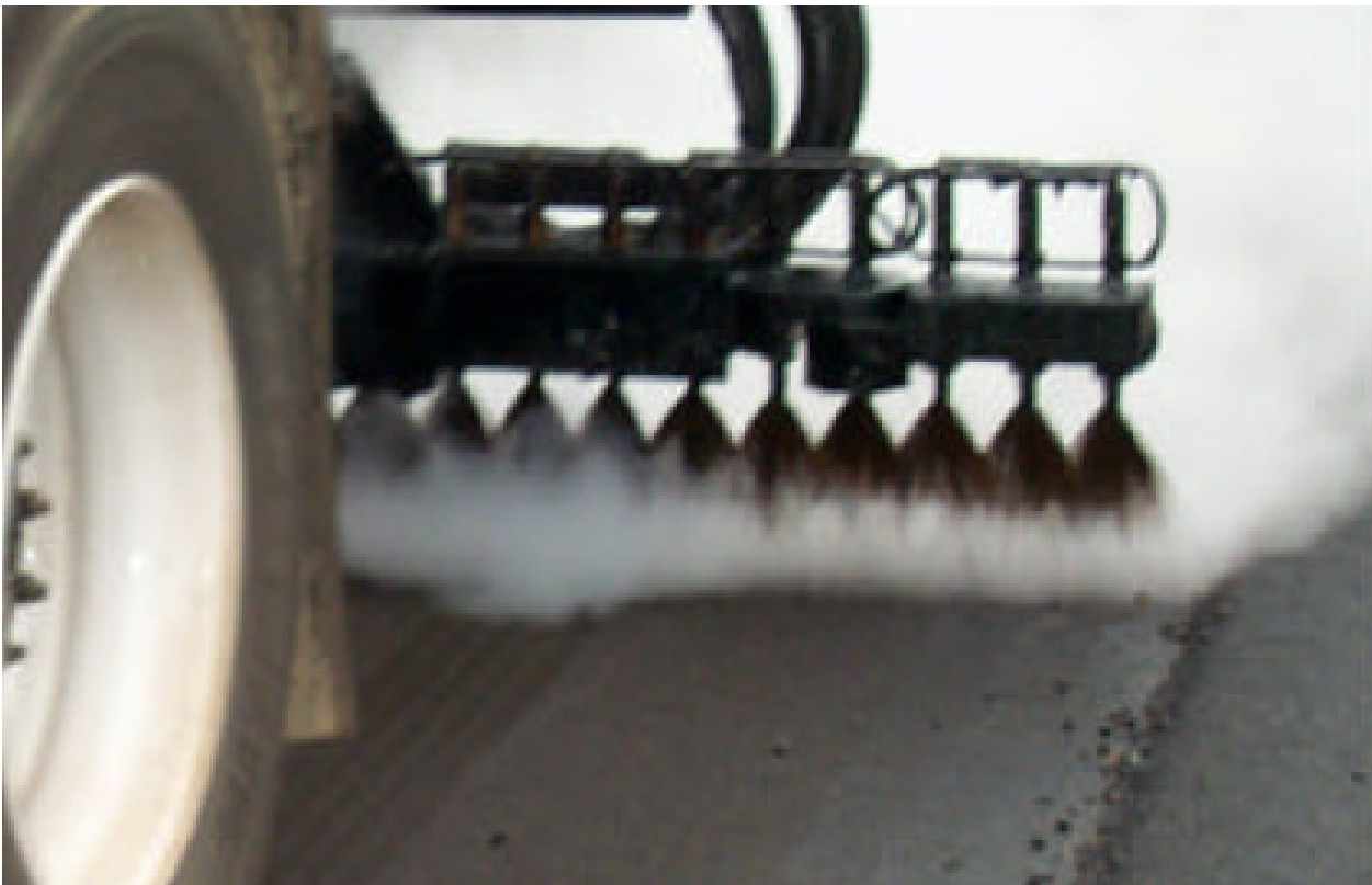
Figure 6. Photo. Proper overlap and spray bar height.
