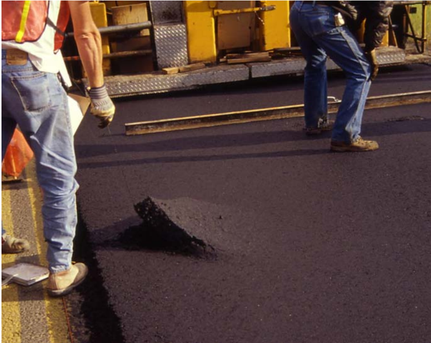
Exhibit 4-5 Obtaining Mixture Sample Prior to Compaction
