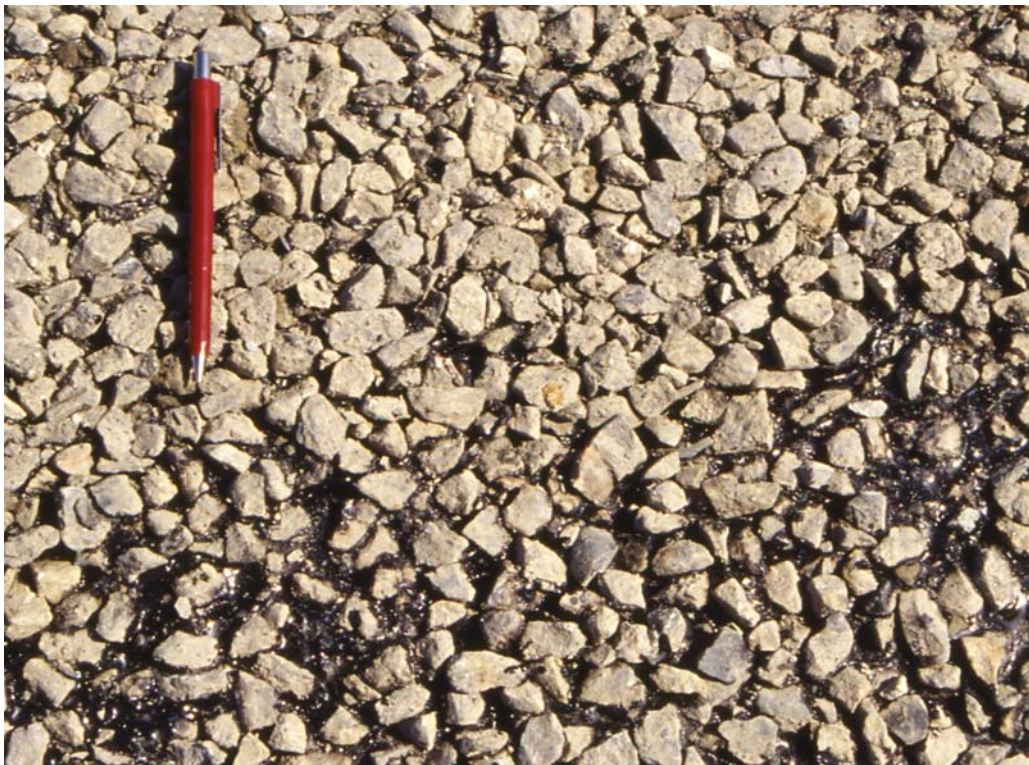
Exhibit 4-14 Completed Chip Seal Surface
