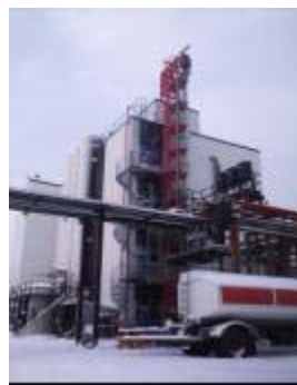
The photo on the left shows an outside view of the solid acid alkylation pilot plant built and operated by the joint venture partners from 2002 to 2004 in Porvoo, Finland. The plant was used to optimize and demonstrate the process. An internal view of the reactors is shown on the right.
