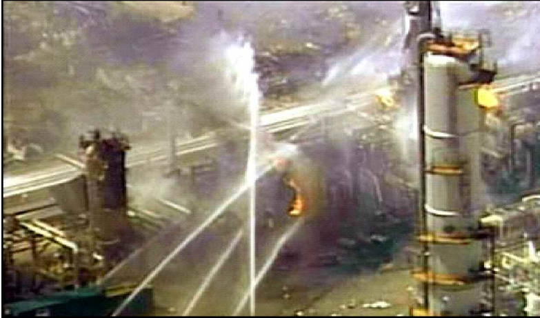
Figure 3. BP Texas City Refinery Fire
