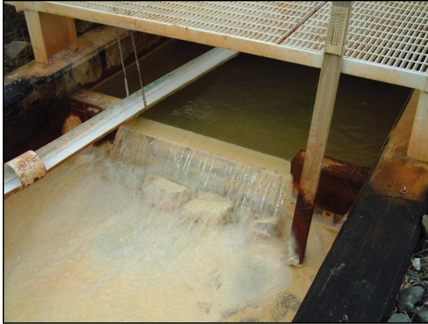
Figure 5. Present Brandy Camp 4-foot broad-crested weir at the treatment plant.
