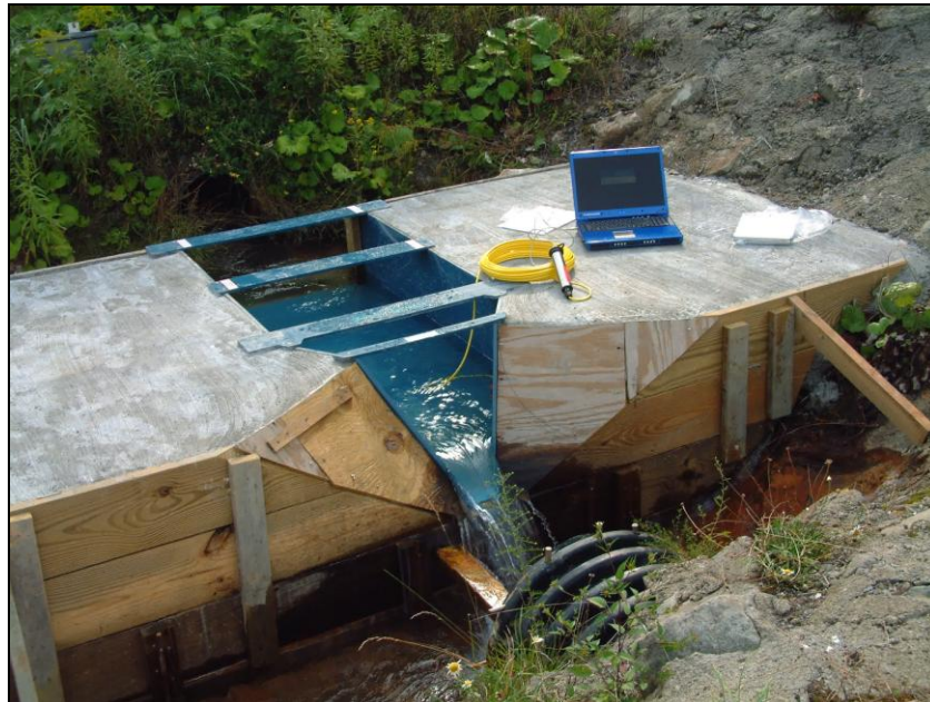
Figure 6. H-type flume installed to measure the overflow discharge rate.
