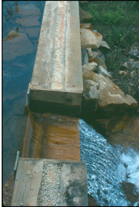
Figure 4. Brandy Camp discharge sharp-crested weir employed for flow monitoring prior to plant construction.
