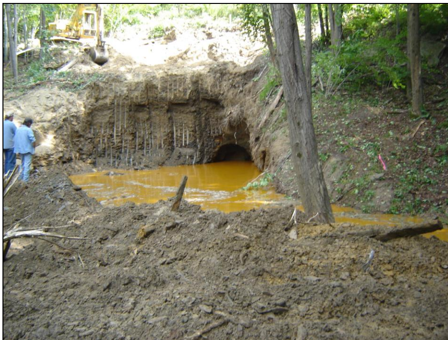
Figure 27. Shawmut Mine portal immediately after excavation.
