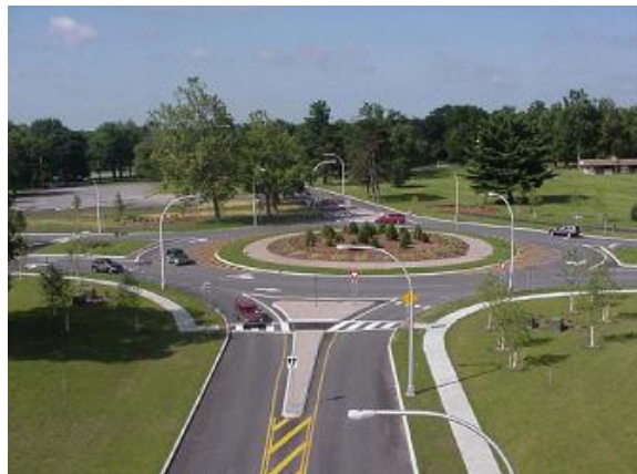
Figure 10. Photograph of a roundabout in New York State, showing the use of pole-mounted lighting (from NYSDOT website).
