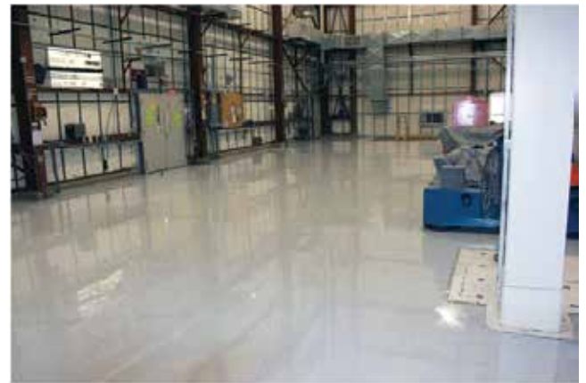
Newly ESD Epoxy Coated Floor in VAB High Bay.
