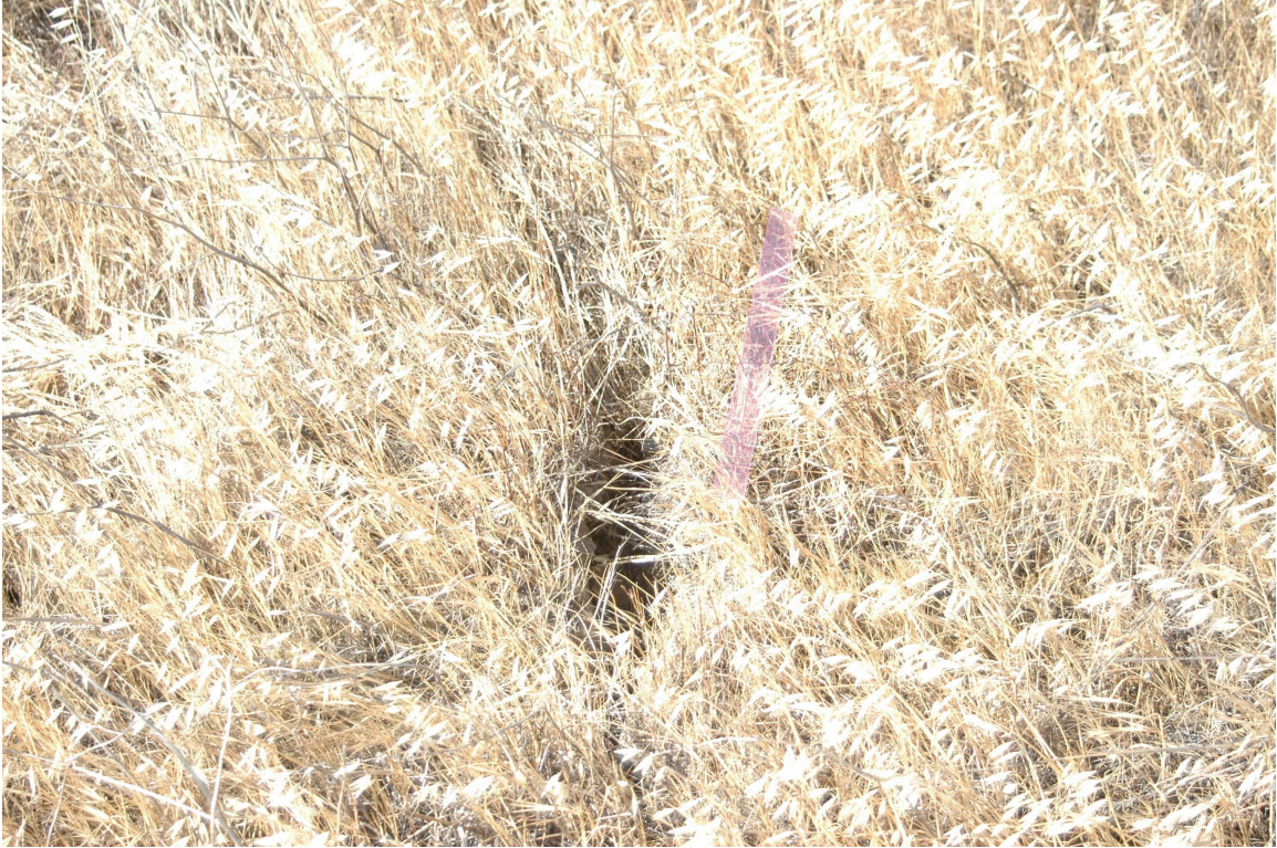
Figure 5 Crack On the Cap
