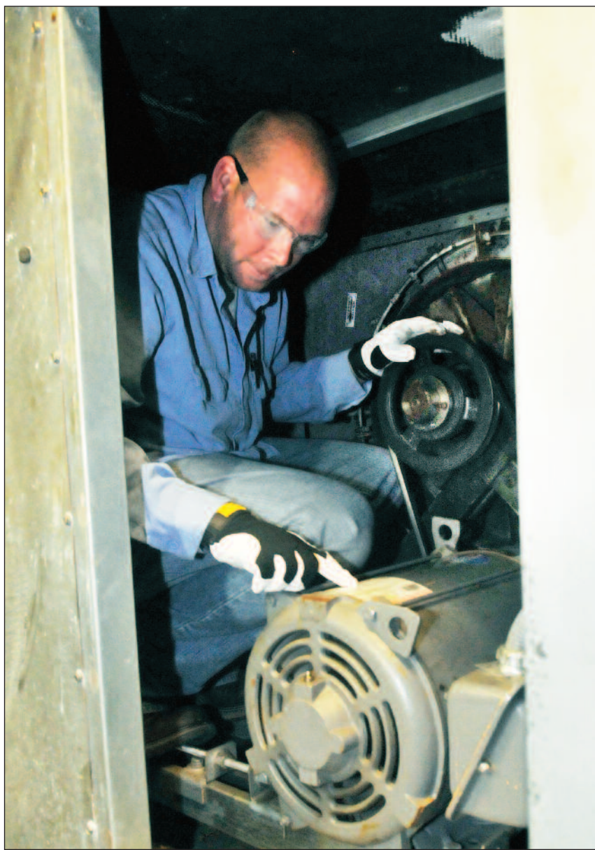
Eric Smith works on a motor and belt inside an air handler.
