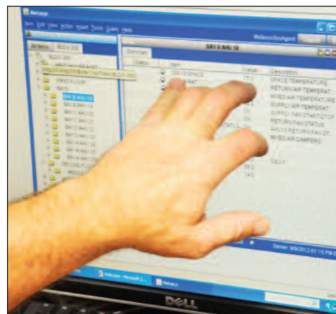
Roy Bowden, 78th Civil Engineer Squadron HVAC shop supervisor, shows how shop employees can access a computer link to buildings to get readings in the Direct Digital Controls Room.
