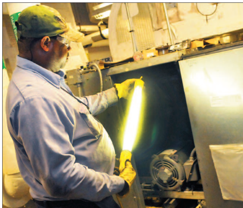
Eric Smith works on a motor and belt inside an air handler.
