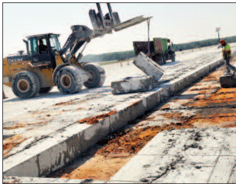
Workers remove concrete slabs from the Runway 33 touchdown zone. Weather permitting, construction is slated for completion next week.
