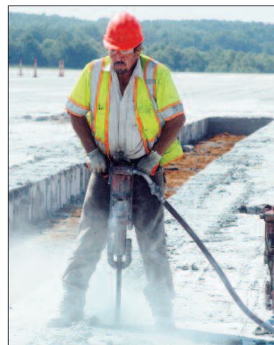
Workers remove concrete slabs from the Runway 33 touchdown zone. Weather permitting, construction is slated for completion next week.
