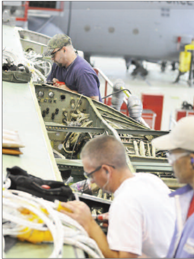
U.S. Air Force photos by SUE SAPP Top to bottom, Jonathan Hampton, Mike Pickens and Sam Wiggins, 402nd Aircraft Maintenance Group, work to attach the main vertical beam into a new C-130 center wing box.
