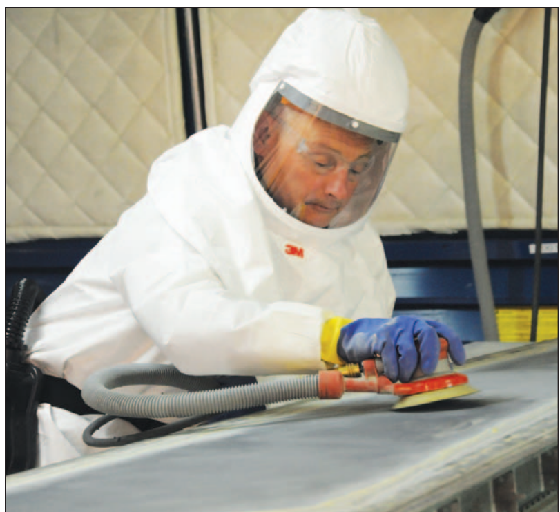
U.S. Air Force photo by RAY CRAYTON Ronnie Gadola, 574th Composite Repair Flight sheet metal mechanic, sands an F-15 torque box assembly in a new sanding booth in Bldg. 169.
