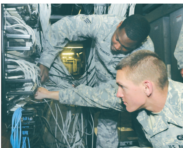
Airman Nicholas Johns, right, and Senior Airman Edward Edwards, 78th Communications Squadron network infrastructure technicians, make the last of 1,300 network switch upgrades in Bldg. 300.
