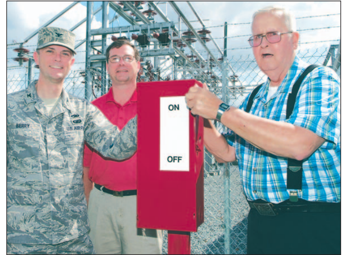
U.S. Air Force photo by GARY CUTRELL Col. Warren Berry, 78th Air Base Wing commander, joins Jim Holten, Georgia Power project manager, and former 78th Civil Engineer Group employee Bill Fowler in flipping the ceremonial first switch on the new electrical substation.
