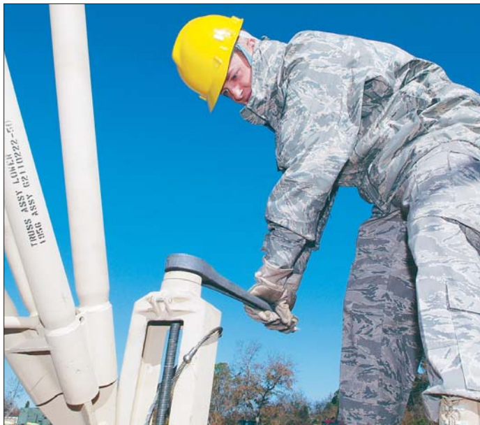
Airman 1st Class David Hunstberger tightens the anchors for the antenna of the ANTRC-170, a Tropospheric Scatter Microwave Radio Terminal.
