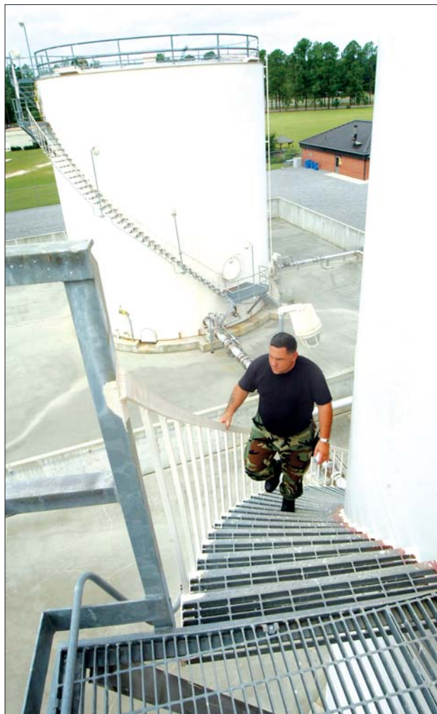
Above, Staff Sgt. Keith Sentak takes the trek up the steps outside of a storage tank to the top.
