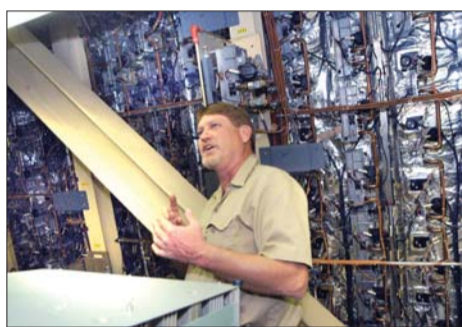
Above from left to right, Two large generators are housed in the PAVE PAWS facility. Charles Haas stands in front of the interior wall of one of the array faces showing all the electrical wiring supporting the arrays. When operating, a light in the control room would tell if the array face was radiated.
