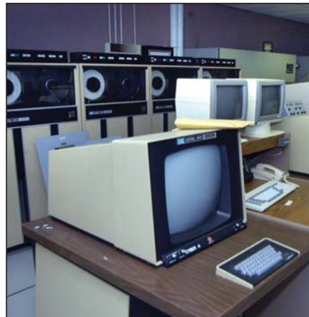
Above, Old equipment used during the peak of the once controlled entry facility, now stands silent in the computer room.
