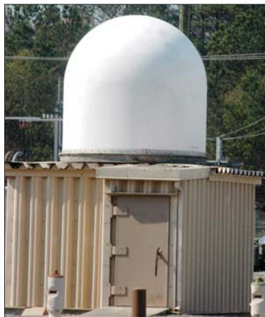
Outside of the PAVE PAWS facility this small building supported the Milstar Satellite Communications System that enabled communication with Air Force Space Command by electro-magnetic pulses.
