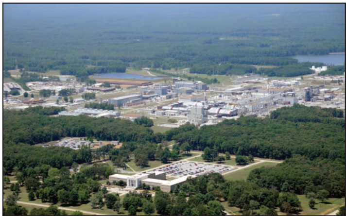
Top, Arnold Engineering Development Center (AEDC) as it appeared during its construction in the 1950s. Below, AEDC in 2008.
