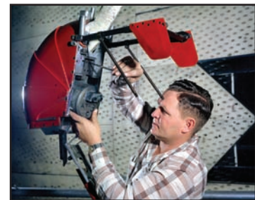
The high-speed crew escape capsule was tested in 16T in 1961.
