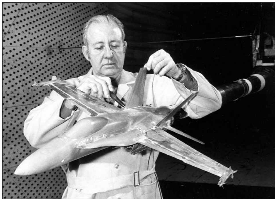
Extensive wind tunnel tests have examined the flight characteristics of the Navy's F/A-18 fighter. In the first phase of the tests, drag measurements were made at simulated flight speeds from Mach 0.6 to 1.55.
