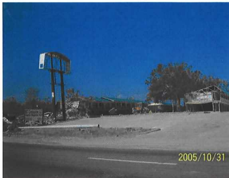
Figure 4.34 Roof Structural Failure on Wood Building
