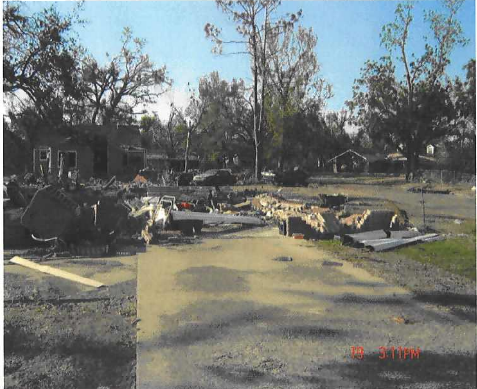
Picture of Foundation (slab) in the Gulf Coast
