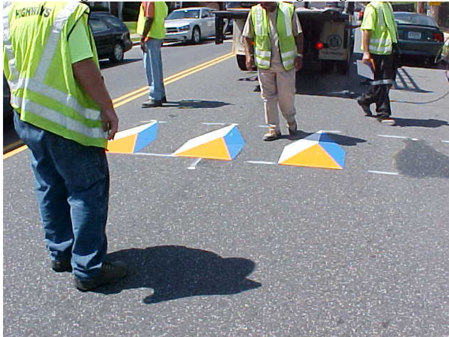
Figure 11. 3-D Pavement Marking Being Installed
