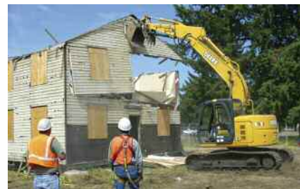
Workers remove a panel from a building at Fort Lewis, Wash., during modular deconstruction. Photo by Rebekah Barker. Date: Feb. 05, 2007. Photo courtesy of US Army from: http://www.army.mil/images/2007/02/05/2394/ .
