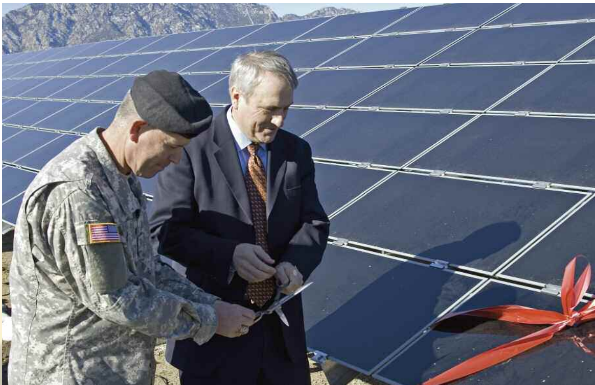
Colorado Governor Bill Ritter Jr and Maj Gen Mark A Graham cut the ribbon on the Army's largest solar array, a 2-megawatt system at Fort Carson that should produce enough power for 540 homes Fort Carson won the Governor's Renewable Energy Award for 2007 for its efforts in the solar array project Photo by Staff Sgt Jim Greenhill Photo courtesy of US Army: www.army.com/news/item/3481 .
