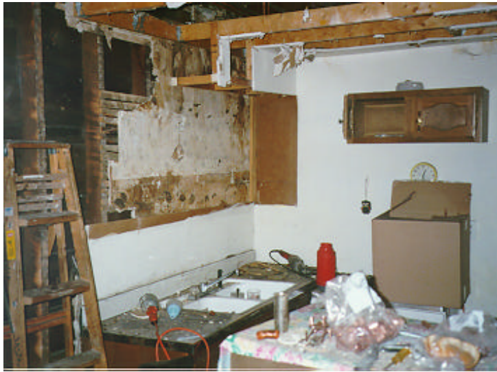
Work behind schedule, Rensselaer, NY
