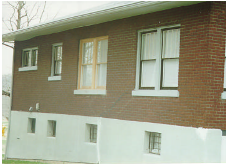
Unpainted new window, Louisville, KY
