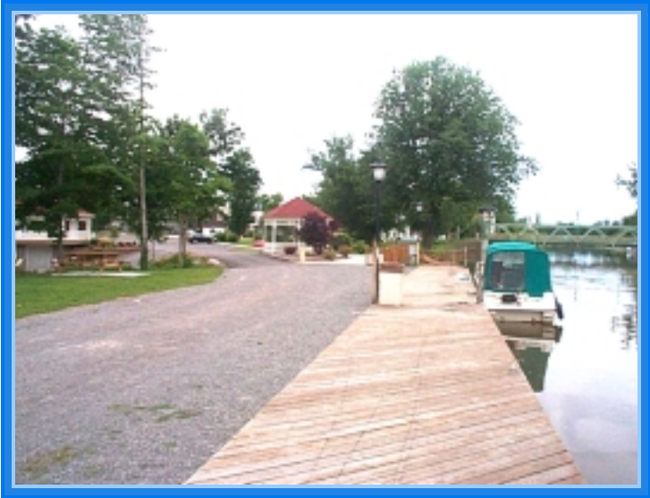
Holley, N.Y. Public Improvements - Canal Wall and Dock.
