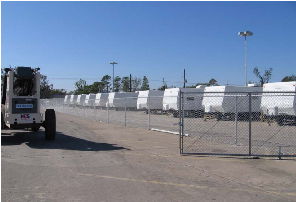
Figure 1 - An Emergency Group Shelter in St. Bernard Parish
