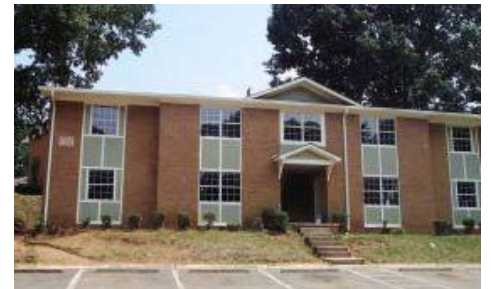
After: The rehabilitated apartments of Flat Shoals.
