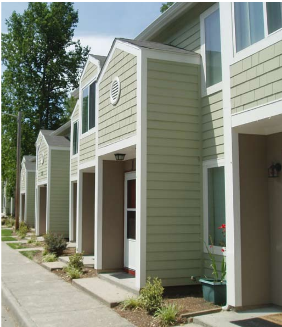
Community Housing Partners recently completed a “green” renovation of Yorktown Square II, which provides housing to low-income residents of Yorktown, Virginia.
