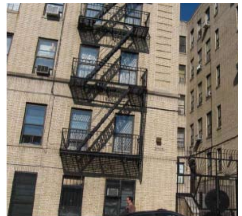
This Bronx project, on Davison Avenue, was part of a portfolio of six, unsubsidized properties rehabilitated by the Fordham-Bedford Community Development Corporation.
