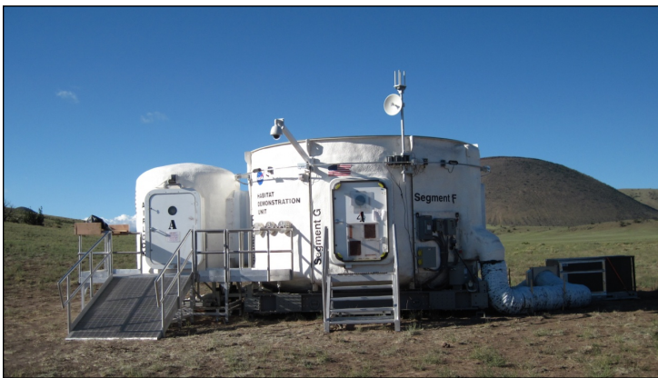
Figure 1. An image of the HDU in front of the SP Mountain. The larger component to the right is the PEM and the smaller structure to the left is the airlock.
