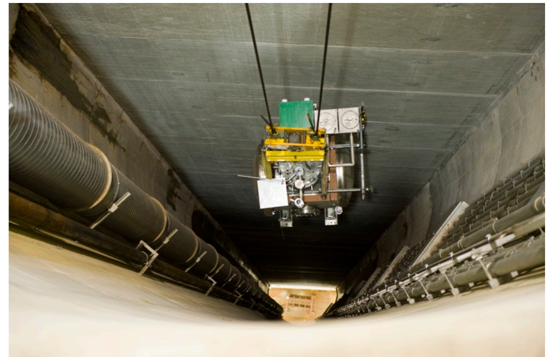
Moving underground (lowering down 350 ft. shaft)
