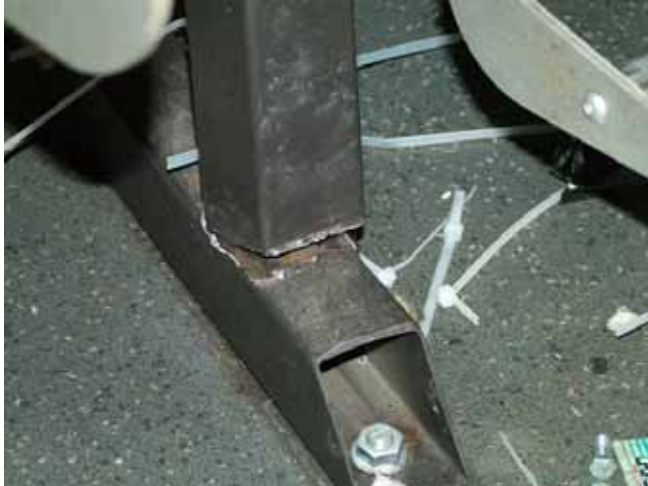
Figure 25 - Damage to the seat mounting hardware
