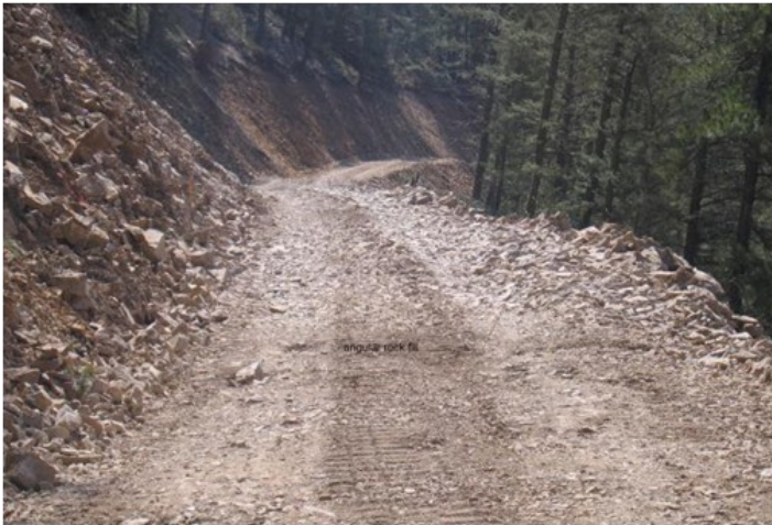
This road will be reclaimed once salvage work is completed.
