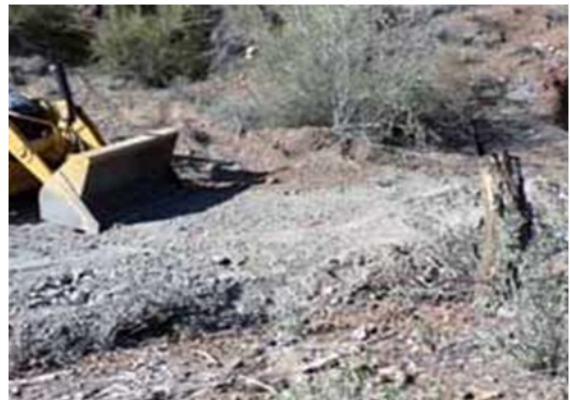
After: Shaft is closed and secured
