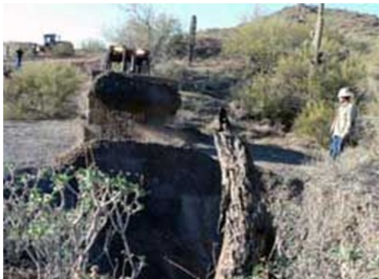
Before: Shaft was more than 100 feet deep.
