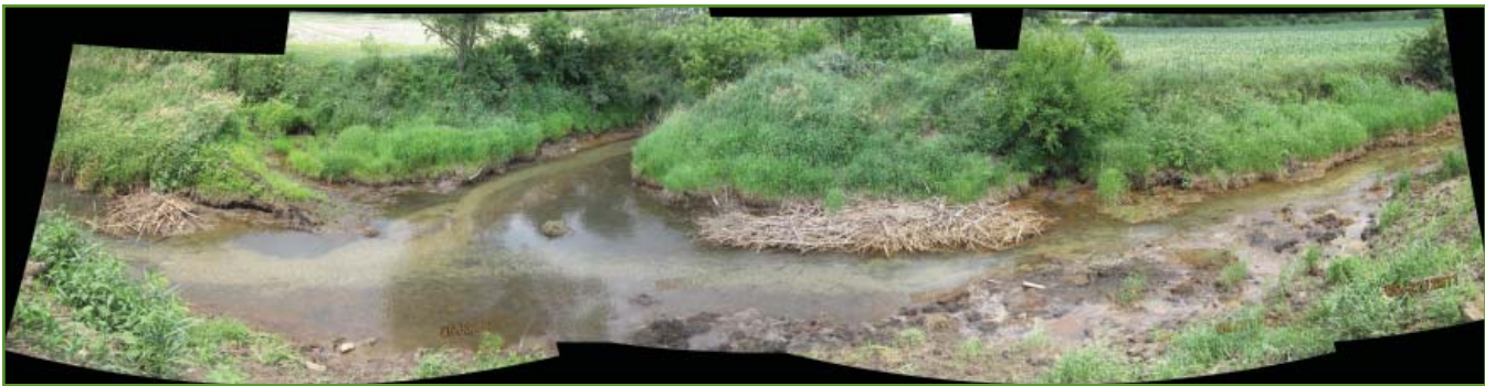
Figure 12: Panoramic view of the junction of Parker-Cobb Ditch and 100West Fork Cobb Ditch, facing northeast. Photo by USACE.
