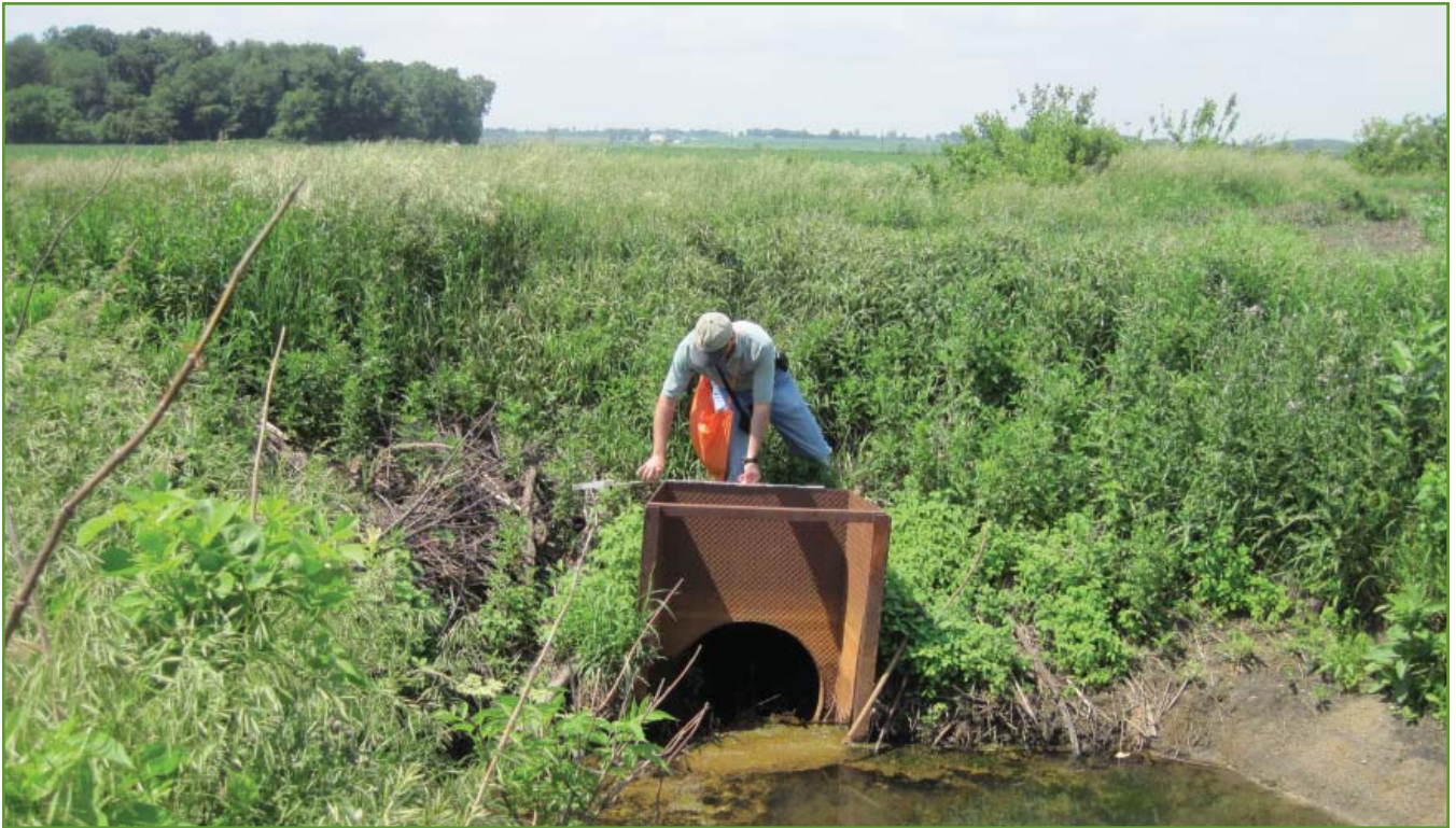
Figure 10. View looking southwest from east bank of West Fork Parker Ditch showing metal headwall and 27-inch (69cm) CMP culvert that extends approximately 40-feet (12 m) and connects with Parker-Cobb Ditch. Photo by USACE.
