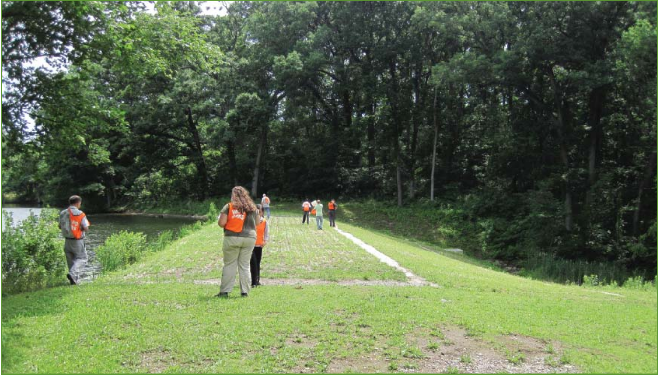
Figure 10. Proffitts Dam on Loomis Lake, looking southwest. Photo taken June 20, 2011 by USACE.
