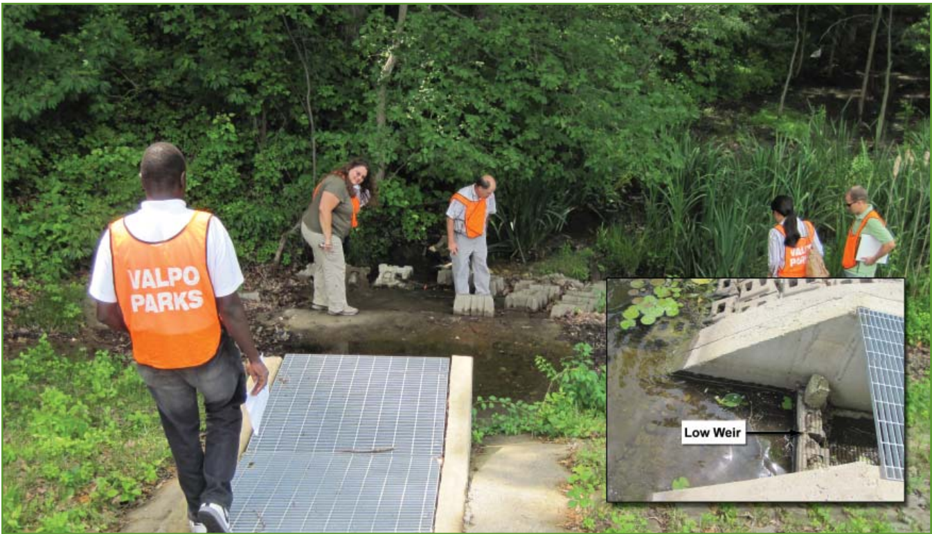
Figure 15. Loomis Lake 3 foot (0.9 m) square (approx.) concrete channel auxiliary spillway to Damon Run, looking downstream; (Inset) Entrance to concrete channel of this auxiliary spillway at Loomis Lake. Photos by USACE
